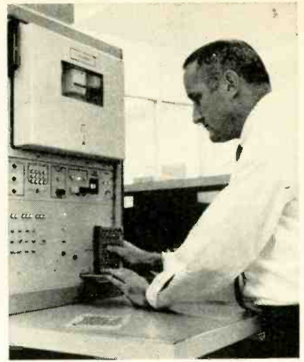
Automatically testing a module "card."
